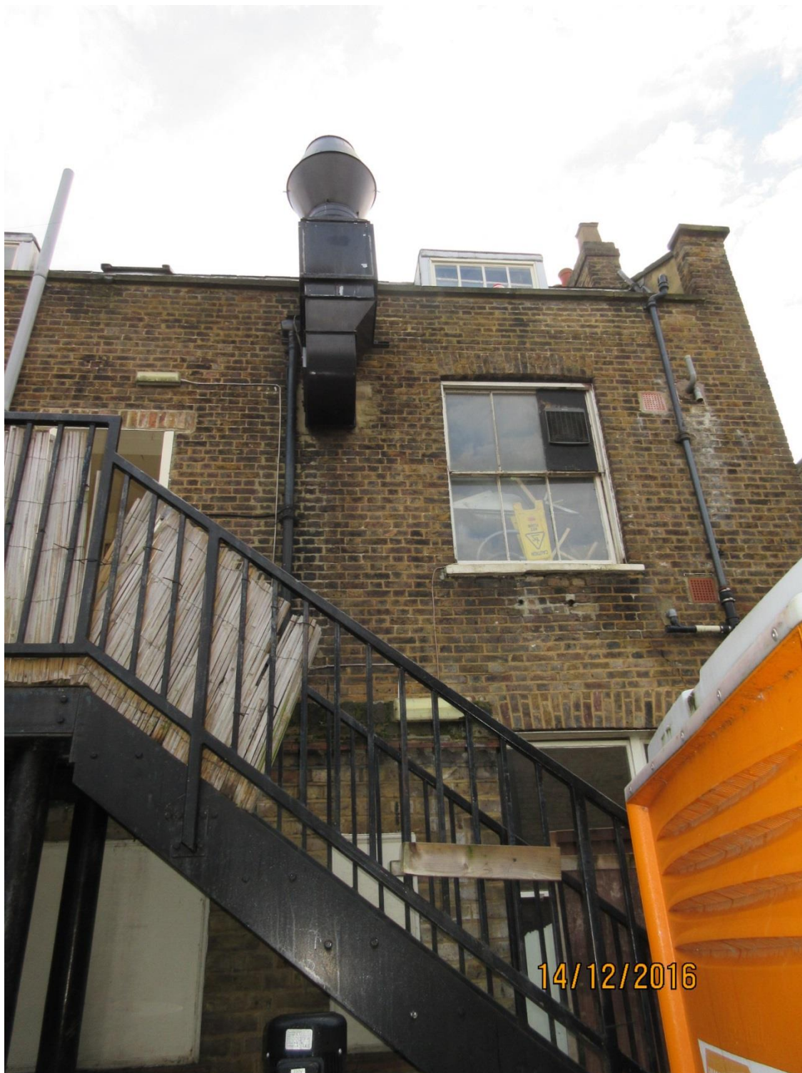
Rear elevation (showing existing flue)
